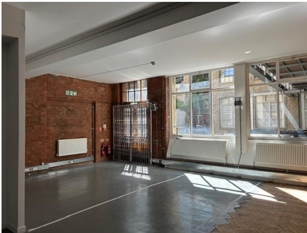
Internal view towards the courtyard
