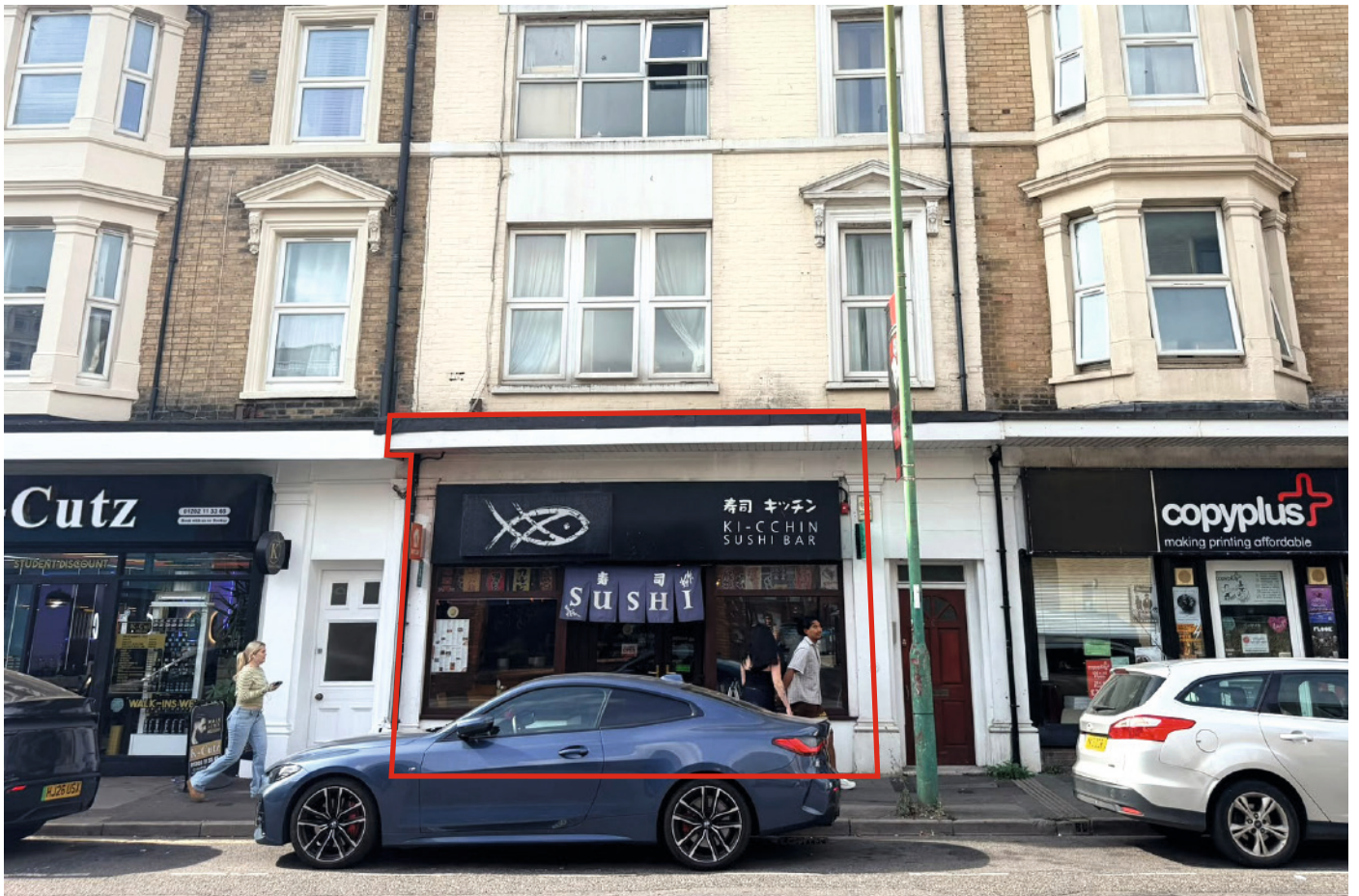
Ground Floor Restaurant
