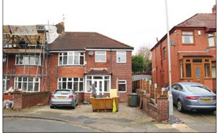
12 Kendal Avenue, Rochdale
