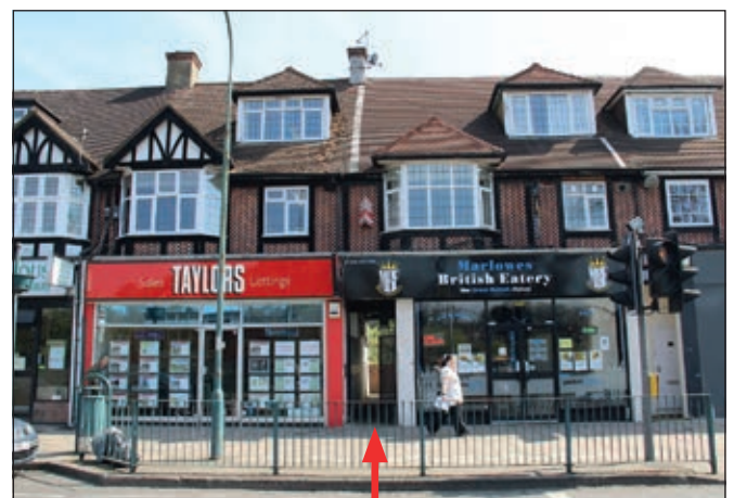
Entrance to No. 19A
