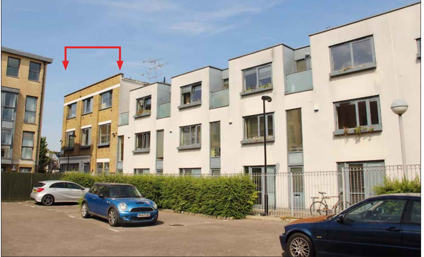
Lower Ground Floor Office
