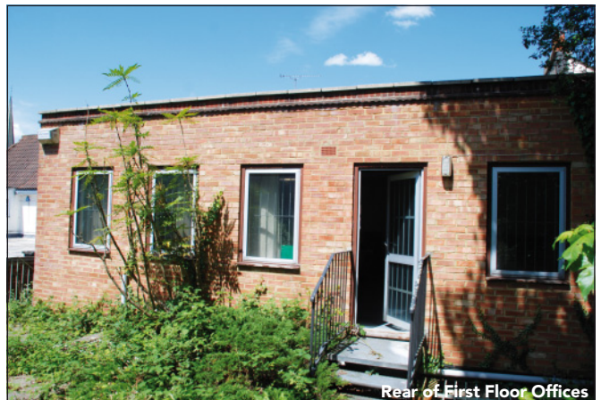
Rear of First Floor Offices
