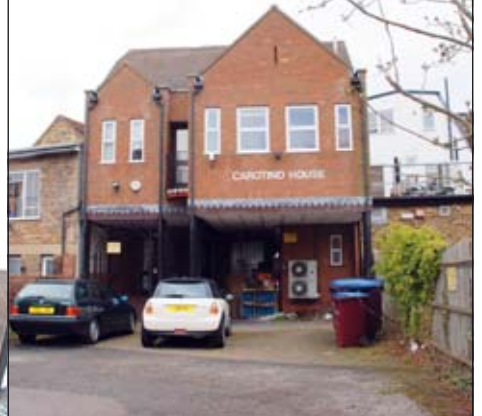
View of Carotino House at rear of property
